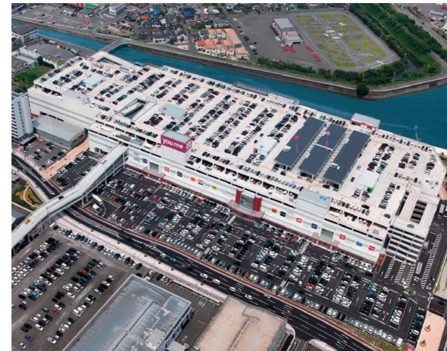
PV panel installed on the rooftop
