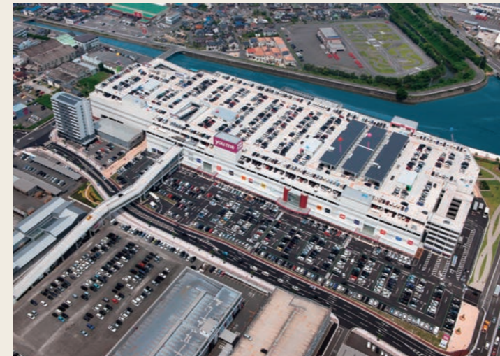
Installation of solar power generation panels on the roof
